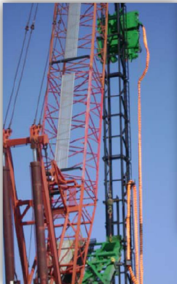
Group and protect hoses on pile driver against stretching and tearing.
